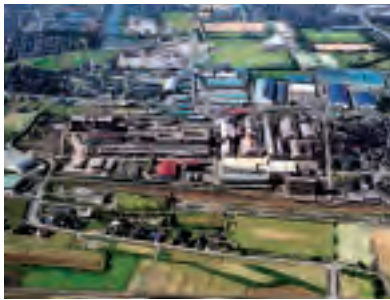
Higashi - Toyama, Steel Plant
