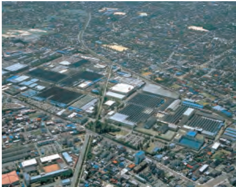
Head Office: Toyama Plant
